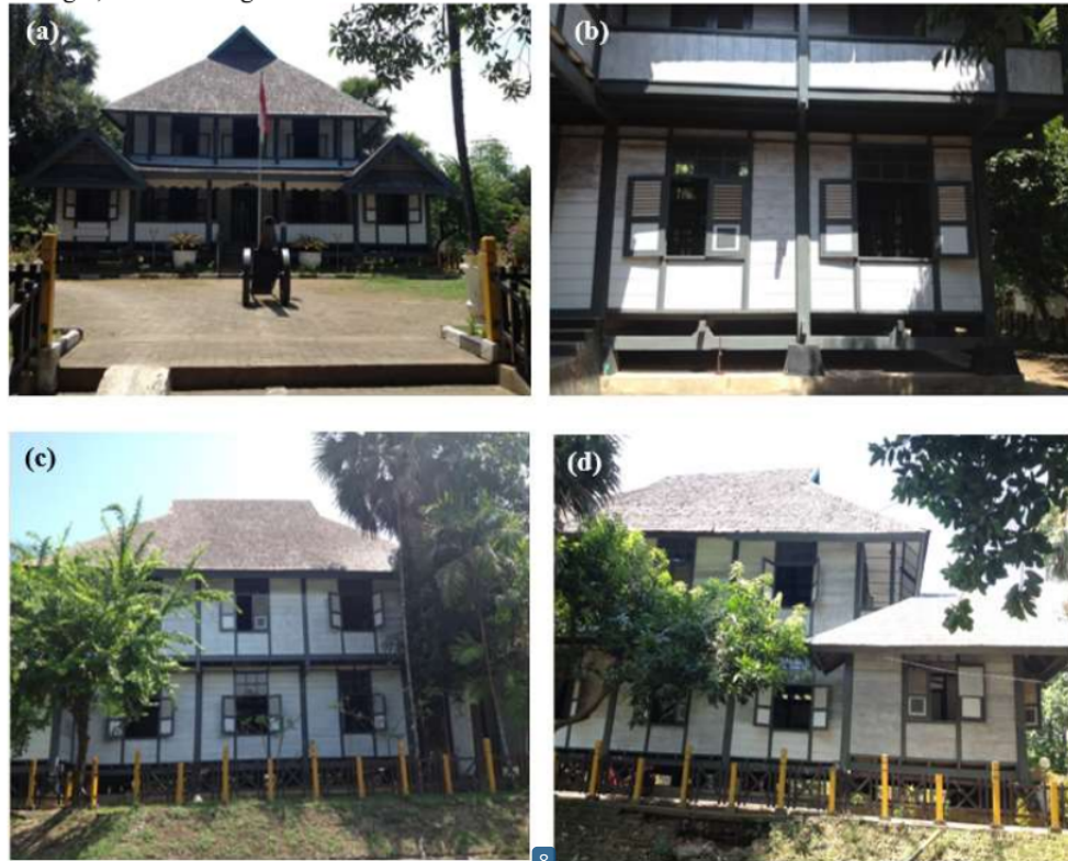
Figure 5. Building surrounding conditions: (a) front, (b) rear, (c) right side, and (d) left side
